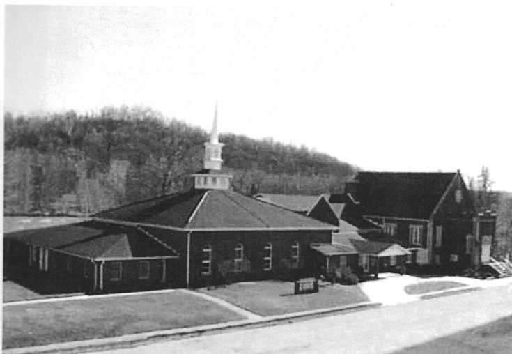
Main Street Baptist Church is located in Point Pleasant, WV.
