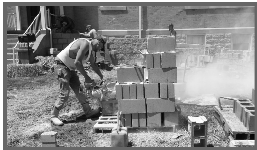
Cutting the blocks on an angle.
