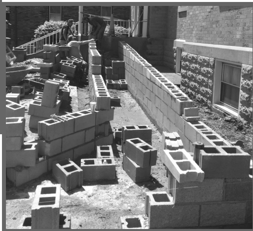
Cutting the blocks on an angle.
